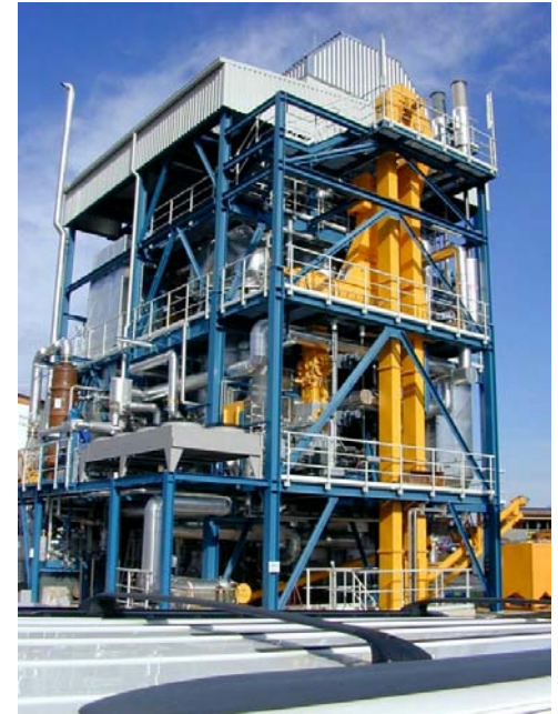
Gasifier in Guessing, Austria (2 MWe, 4.5 MWth)
