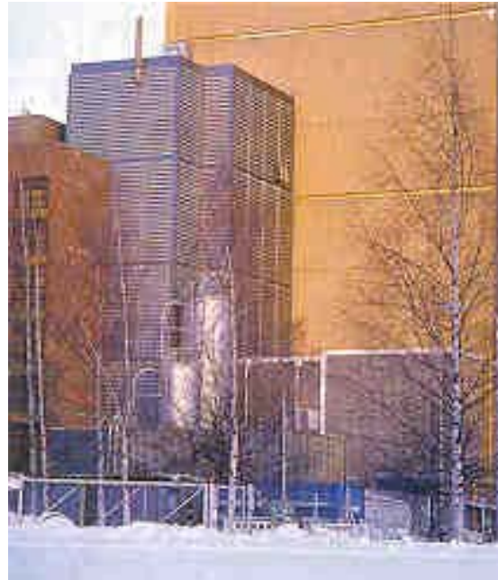
Gasifier at the Kymijävi power plant, Finland (60 MWth)
